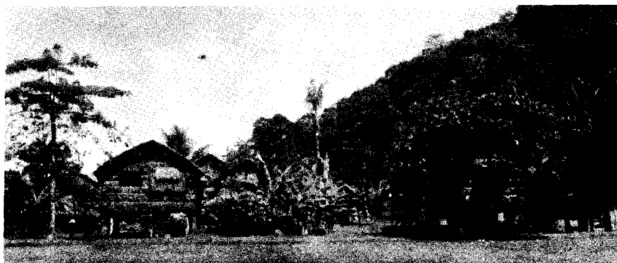
The inland portion of M'buke village.
